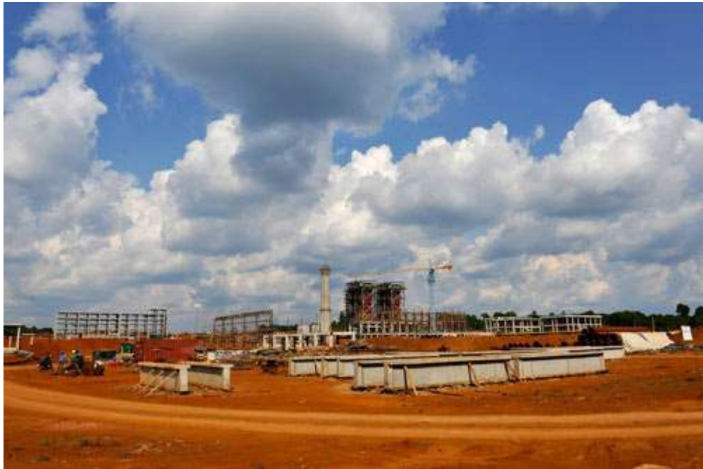
Fig 8. Nhan Co alumina plant building site, October 2013
